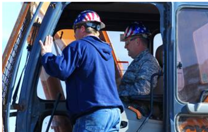
Col. Brad Webb, 1st Special Operations Wing commander, knocks the first blow to the building that formerly housed the 20th Special Operations Squadron and wing plans and programs in a demolition Dec. 6. A new crash/rescue facility for the 1st Special Operations Civil Engineer Squadron Fire Emergency Services Flight will be built at the site. (U.S. Air Force photo/Airman 1st Class Jason Epley)
